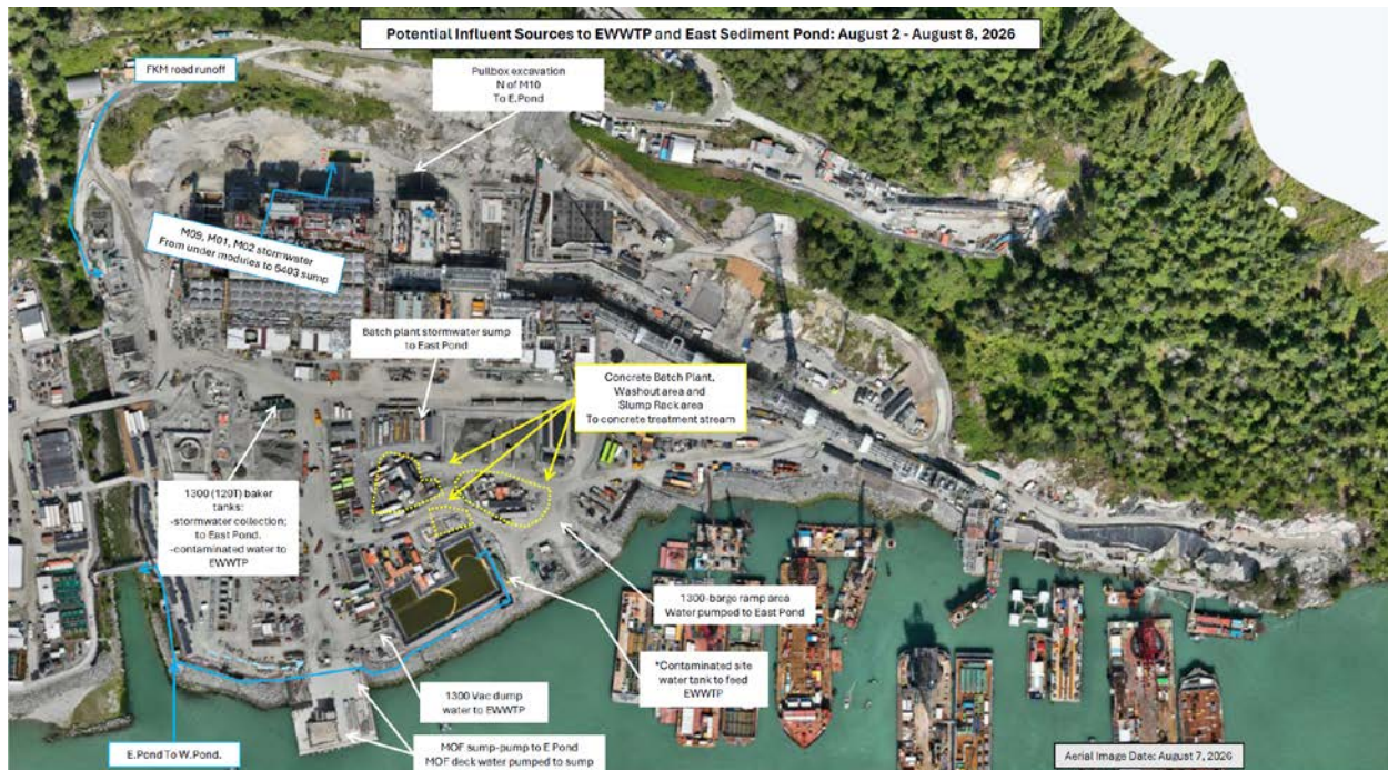
Figure 2: East Catchment contact water management facilities (August 2 – 8).
