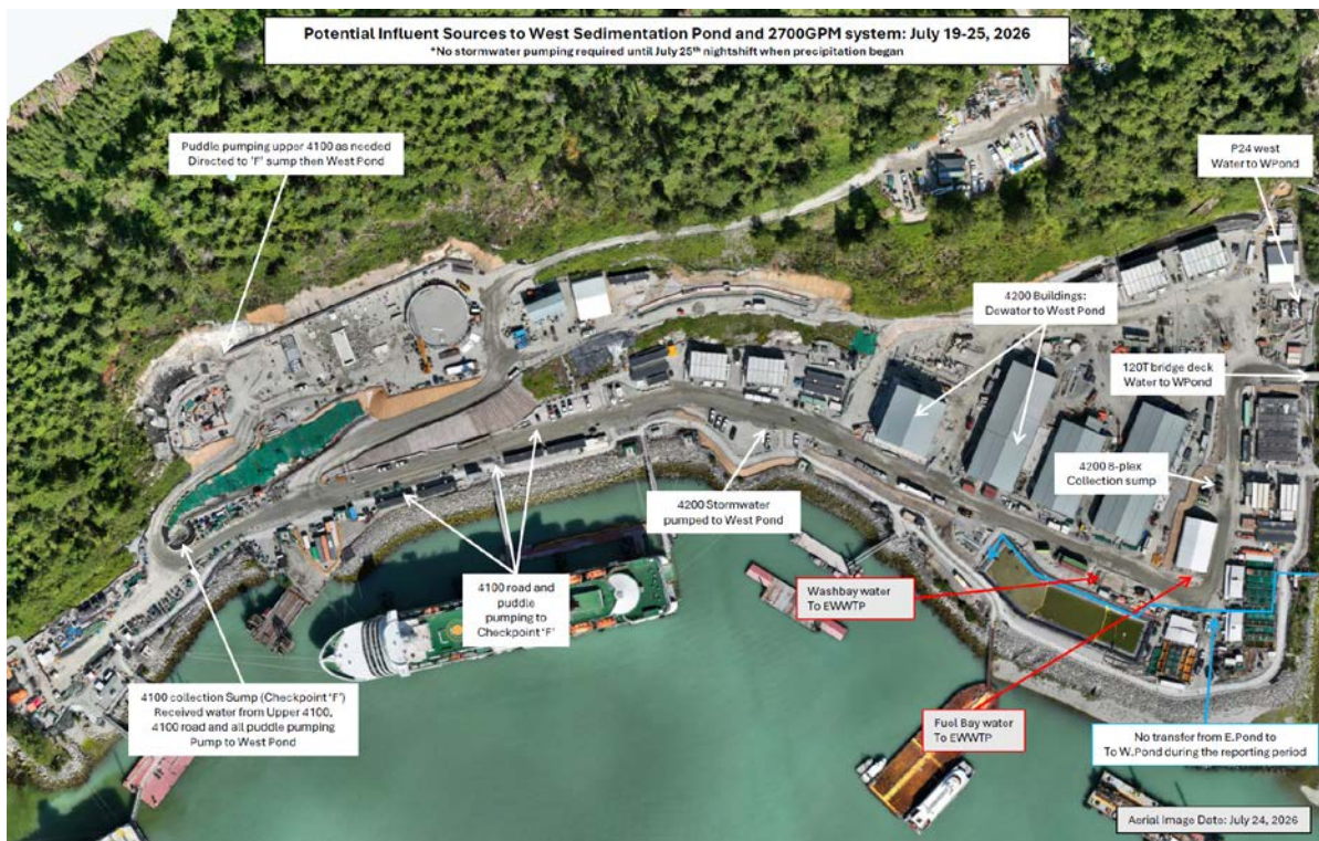
Figure 3: West Catchment contact water management facilities (July 19 - 25).
