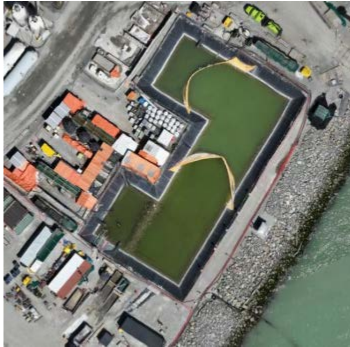
Figure 4: Aerial view of the East Sedimentation Pond (June 19, 2026). The East WWTP is located on the left side of the pond.
