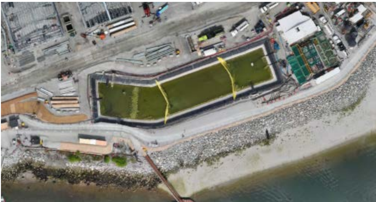
Figure 5: Aerial view of the West Sedimentation Pond (May 1, 2026).
