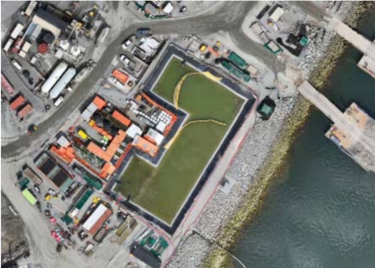
Figure 4: Aerial view of the East Sedimentation Pond (May 1, 2026). The East WWTP is located on the left side of the pond.
