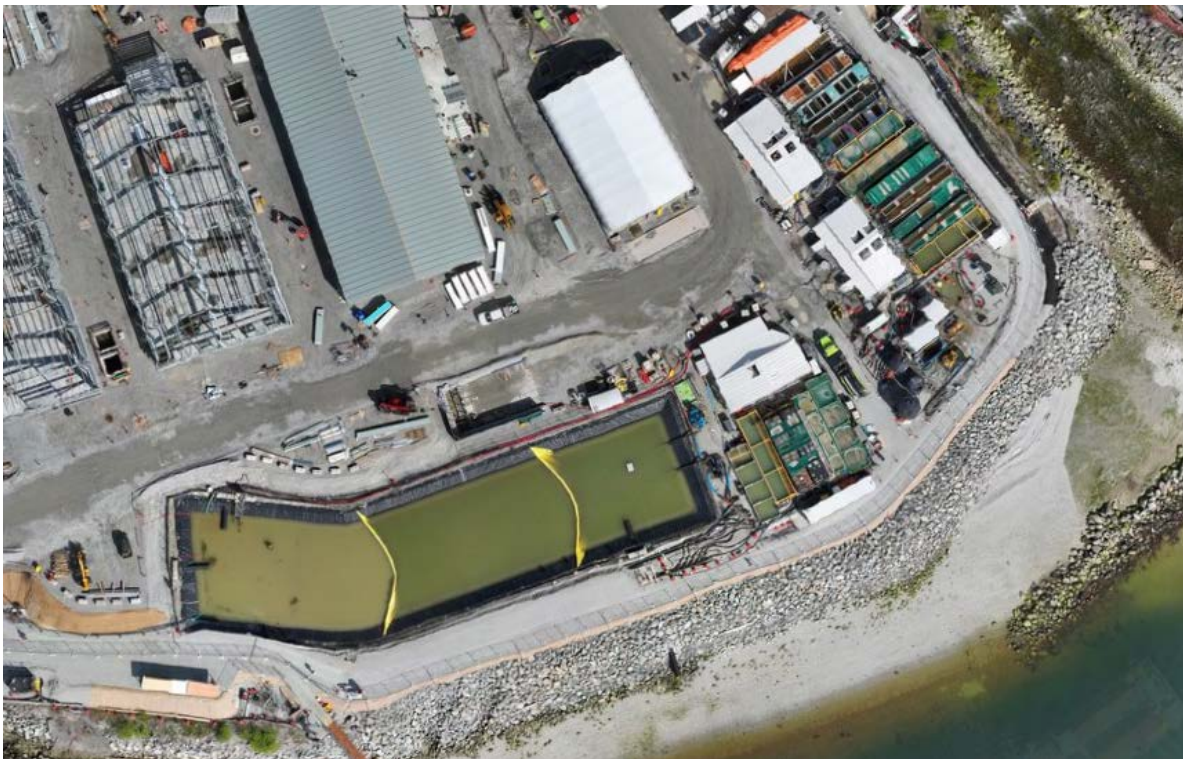
Figure 5: Aerial view of the West Sedimentation Pond (April 17, 2026).
