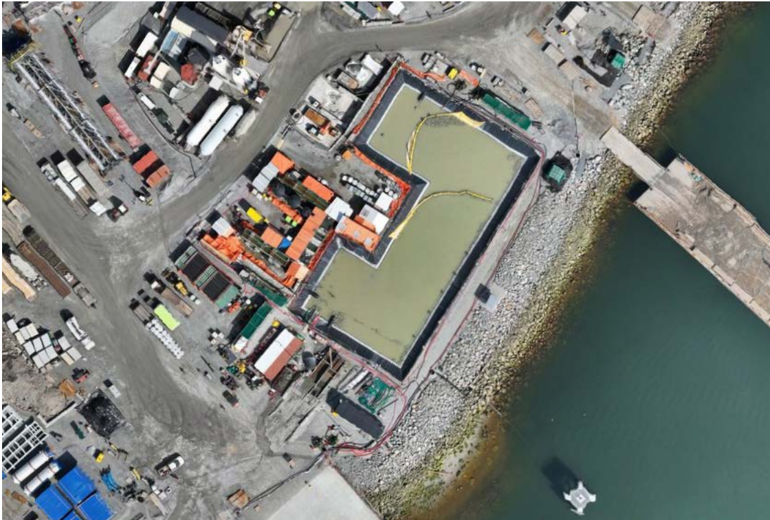
Figure 4: Aerial view of the East Sedimentation Pond (April 17, 2026). The East WWTP is located on the left side of the pond.
