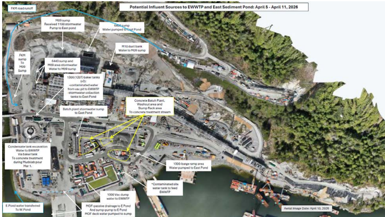
Figure 2: East Catchment contact water management facilities (April 5 – 11).
