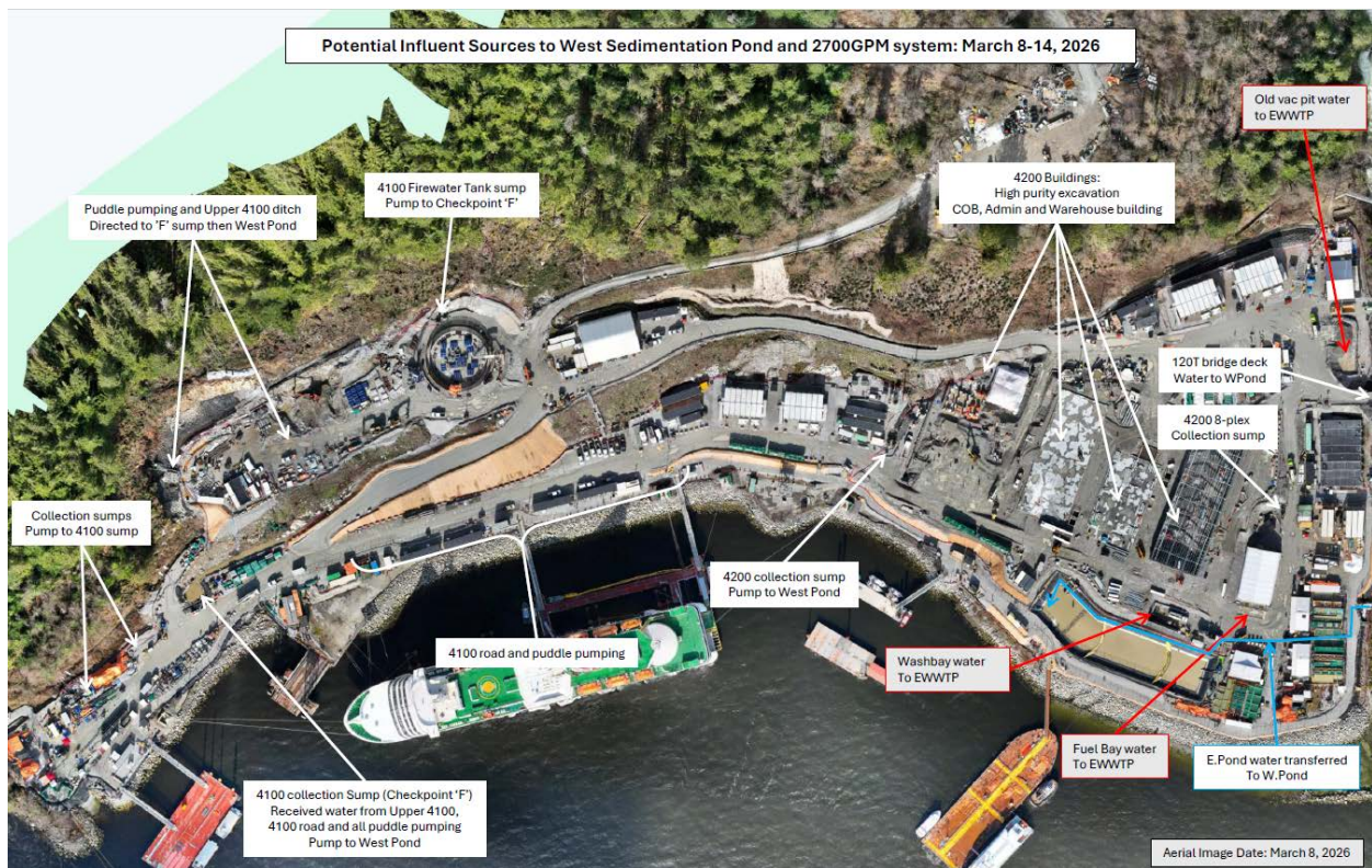
Figure 3: West Catchment contact water management facilities (March 8 – 14).
