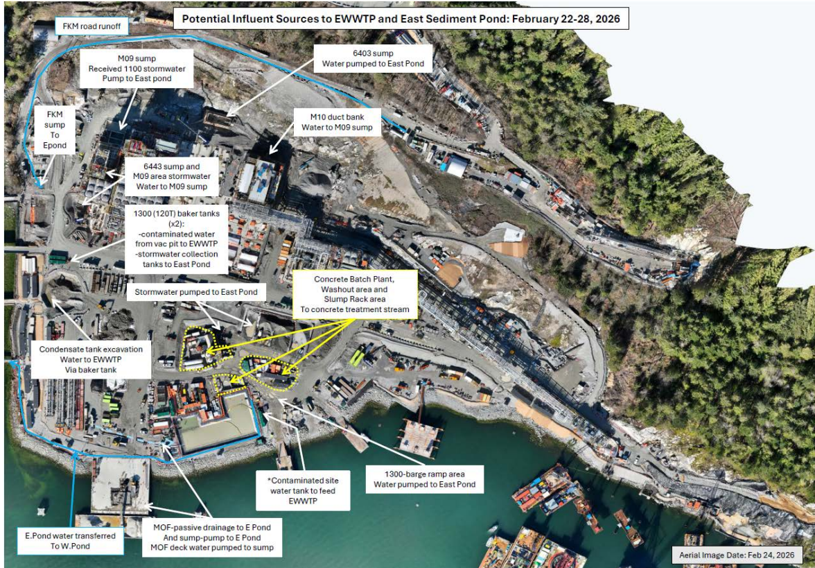
Figure 2: East Catchment contact water management facilities (February 22 – 28).
