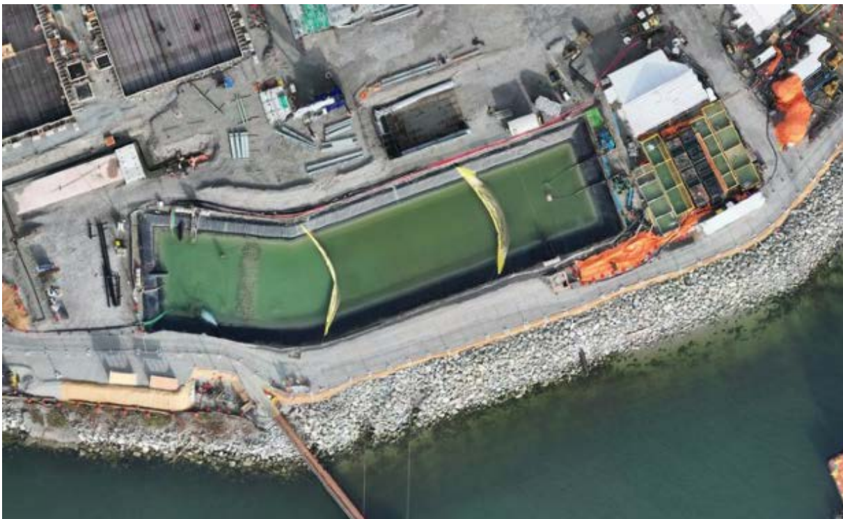
Figure 5: Aerial view of the West Sedimentation Pond (February 6, 2026).
