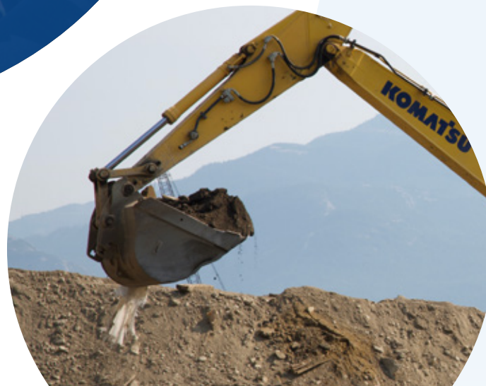
Contaminated Soil Removal
