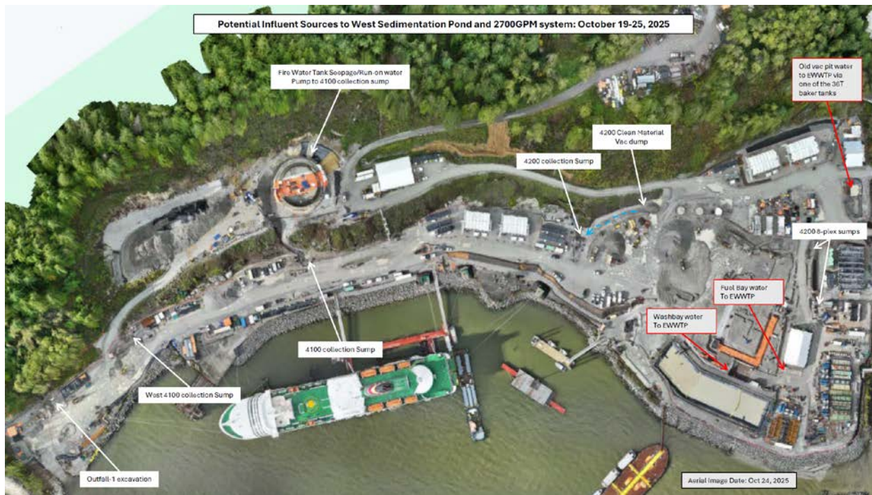
Figure 3: West Catchment contact water management facilities (October 19 – 25).
