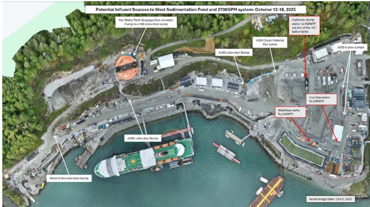
Figure 3: West Catchment contact water management facilities (October 12 – 18).
