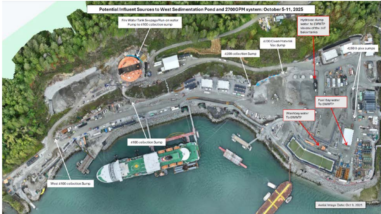
Figure 3: West Catchment contact water management facilities (October 5 – 11).
