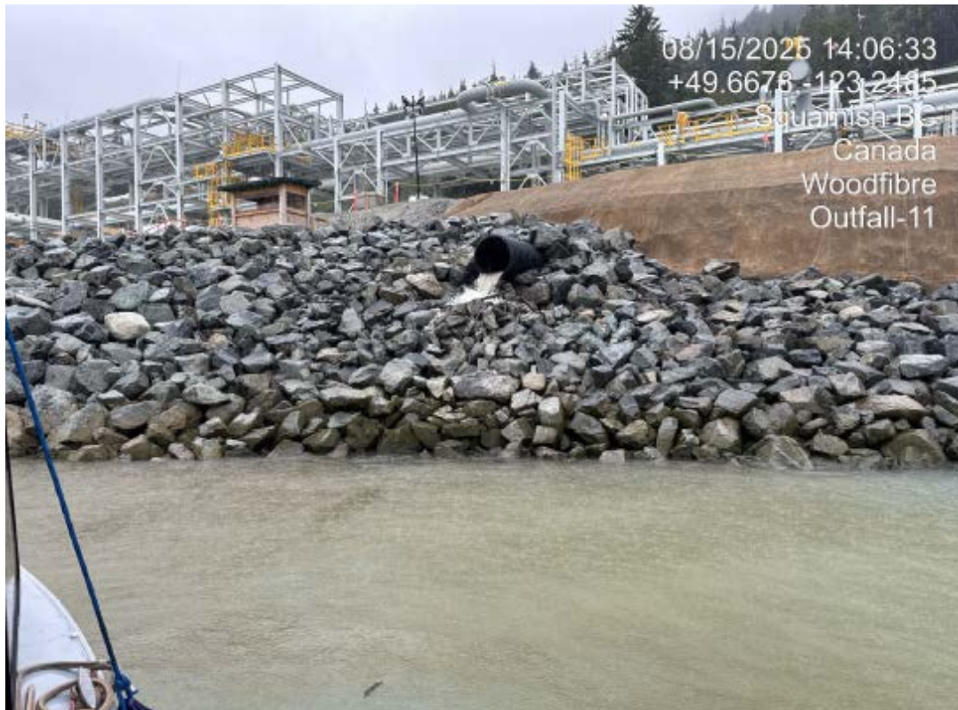
Figure 6: Turbid East Creek water discharging from the OUT-11 culvert on August 15, 2025. Site staff report that the turbid water originated from the upstream reaches of East Creek, outside the LNG export facility construction area.
