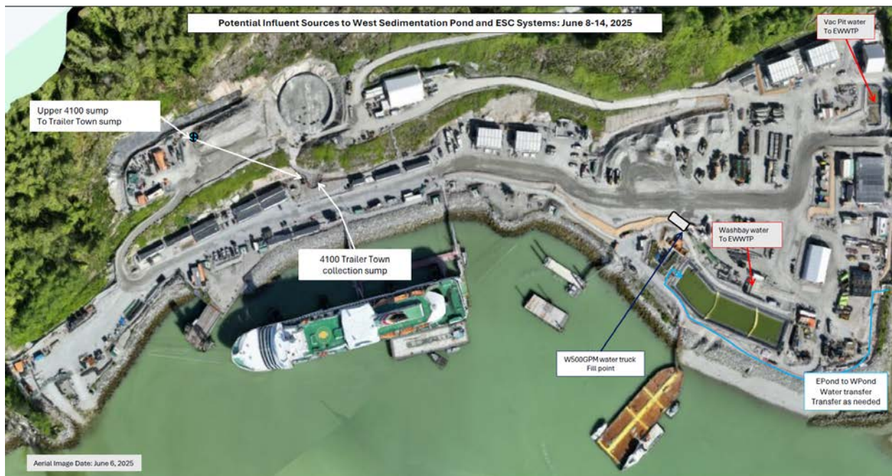
Figure 3: West Catchment contact water management facilities (June 8 – 14).
