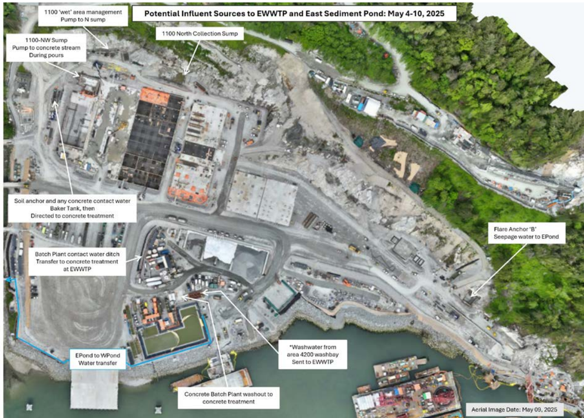
Figure 2: East Catchment contact water management facilities (May 4 – May 10).
