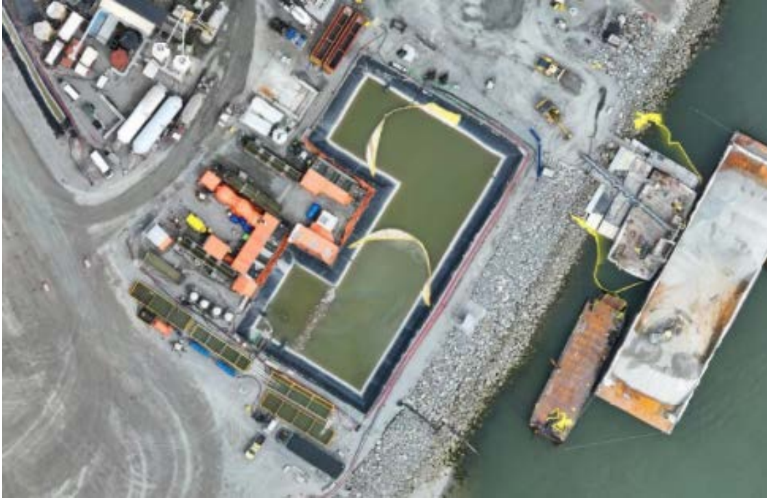
Figure 4: Aerial view of the East Sedimentation Pond (May 9, 2025). The East WWTTP is located on the left side and the E500GPM TSS settling system is situated along the bottom edge of the pond.
