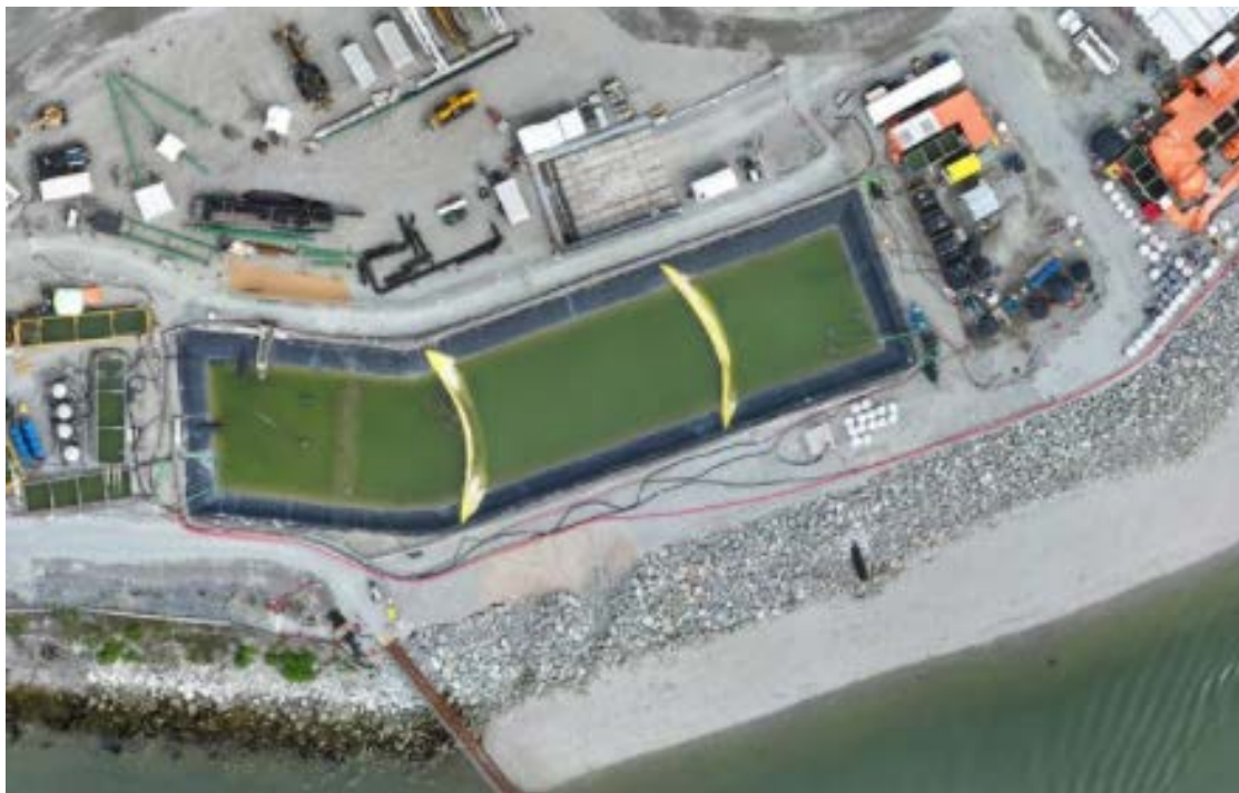
Figure 5: Aerial view of the West Sedimentation Pond (May 9, 2025). The TSS settling systems are located to the left (W500GPM) and right (ESC) of the pond.
