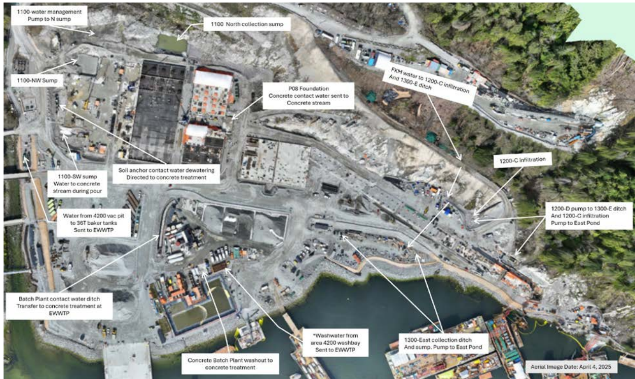
Figure 2: East Catchment contact water management facilities (March 30 – April 5).
