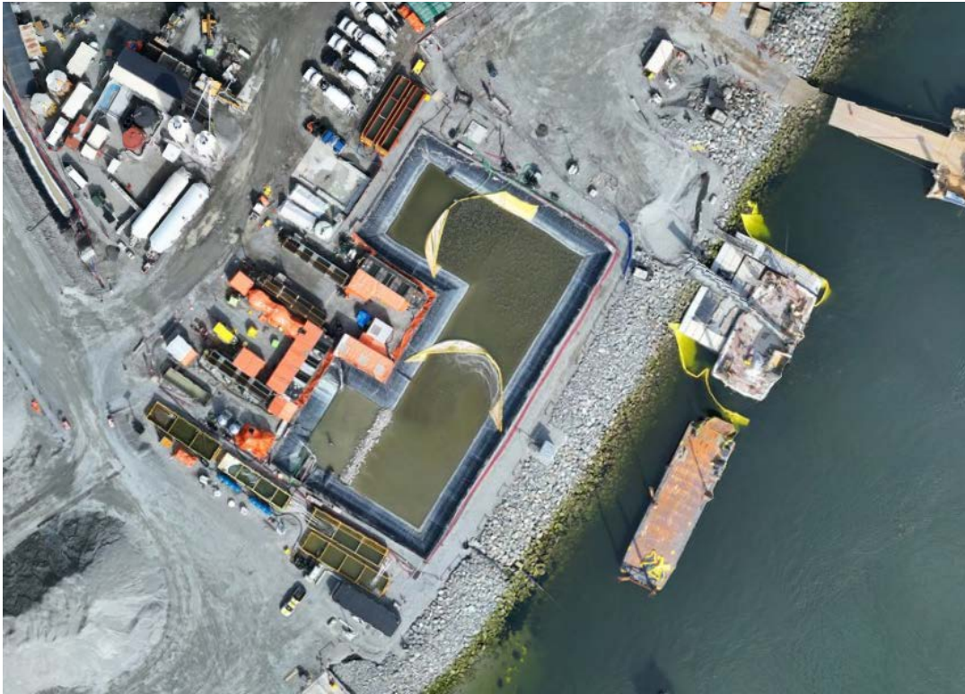
Figure 4: Aerial view of the East Sedimentation Pond (April 4, 2025). The East WWTP is located on the left side and the E500GPM TSS settling system is situated along the bottom edge of the pond.
