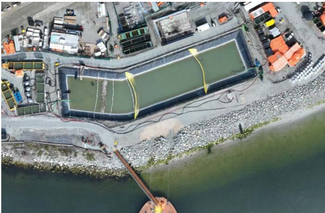
Figure 5: Aerial view of the West Sedimentation Pond (April 4, 2025). The TSS settling systems are located to the left (W500GPM) and right (ESC) of the pond.
