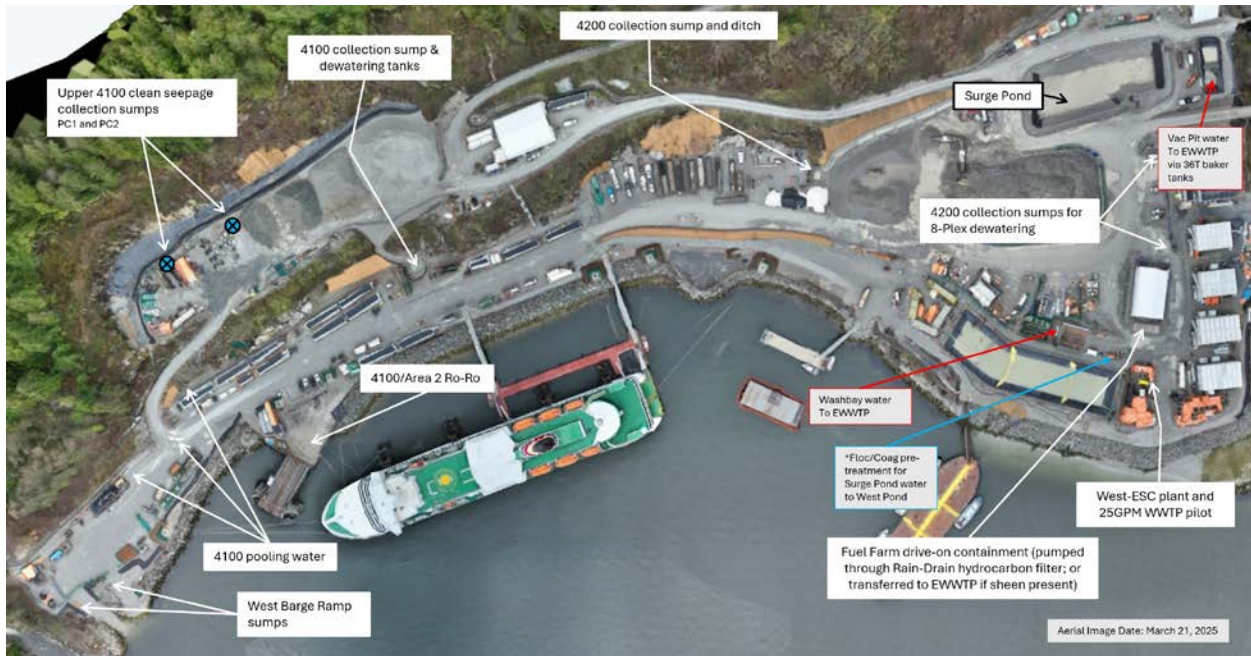
Figure 3: West Catchment contact water management facilities (March 23 – 29).
