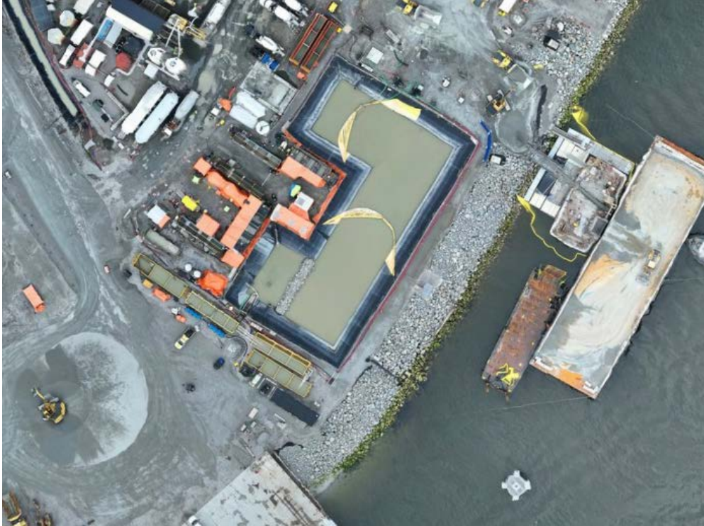
Figure 4: Aerial view of the East Sedimentation Pond (March 29, 2025). The East WWTP is located on the left side and the E500GPM TSS settling system is situated along the bottom edge of the pond.
