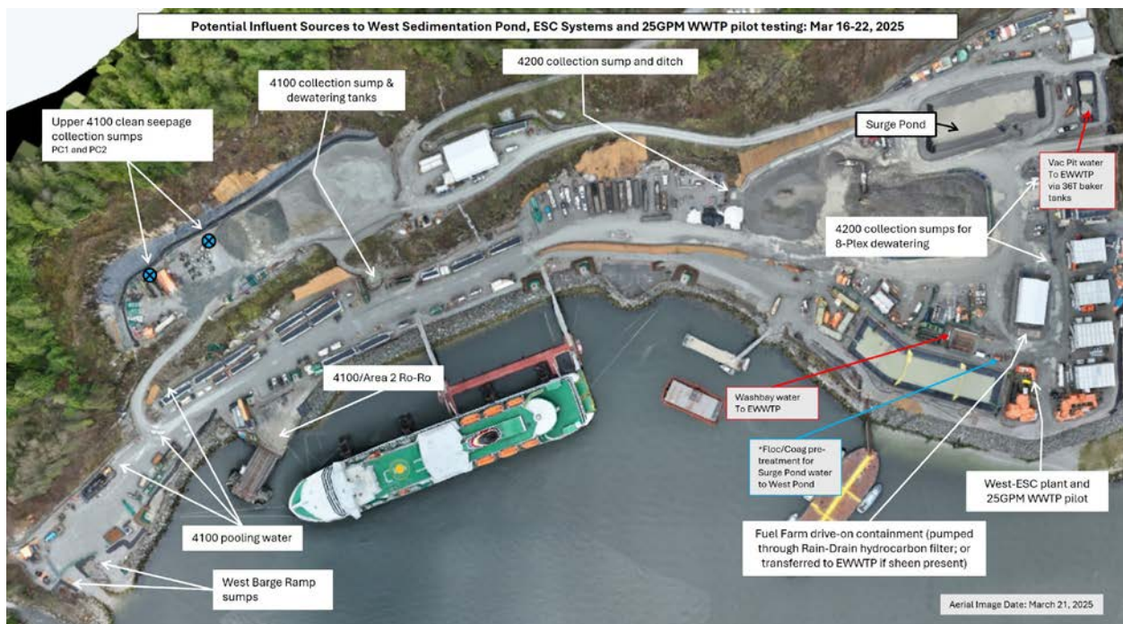
Figure 3: West Catchment contact water management facilities (March 16 – March 22).
