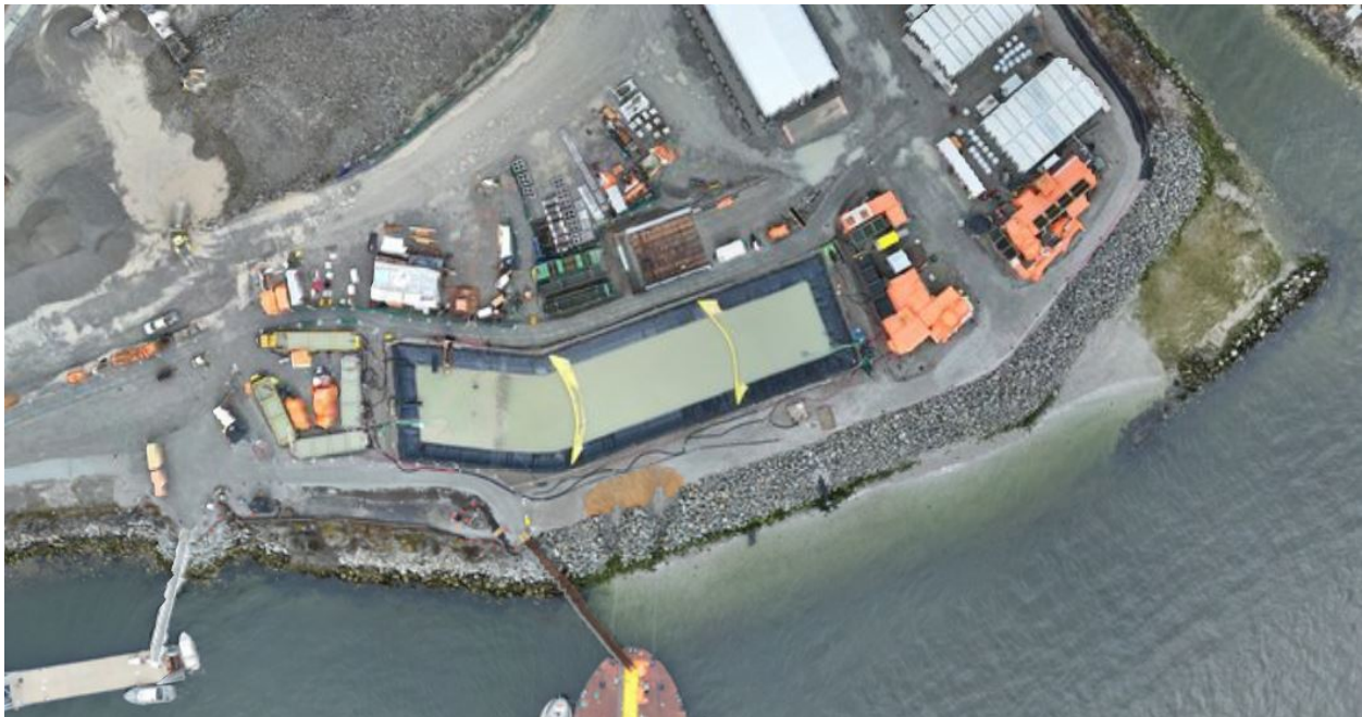
Figure 5: Aerial view of the West Sedimentation Pond (March 21, 2025). The TSS settling systems are located to the left (W500GPM) and right (ESC) of the pond.
