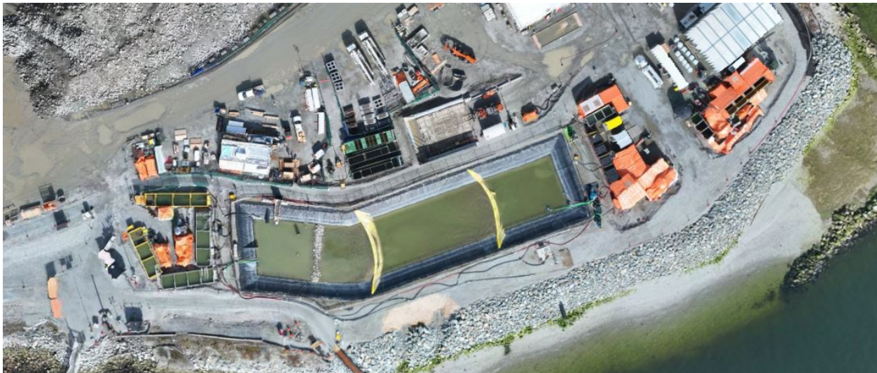
Figure 5: Aerial view of the West Sedimentation Pond (March 14, 2025). The TSS settling systems are located to the left (W500GPM) and right (ESC) of the pond.
