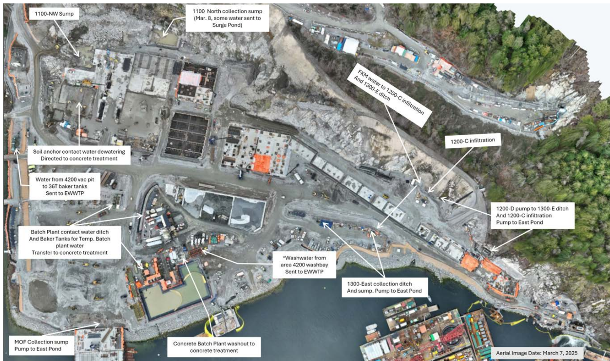
Figure 2: East Catchment contact water management facilities (March 2 – March 8).
