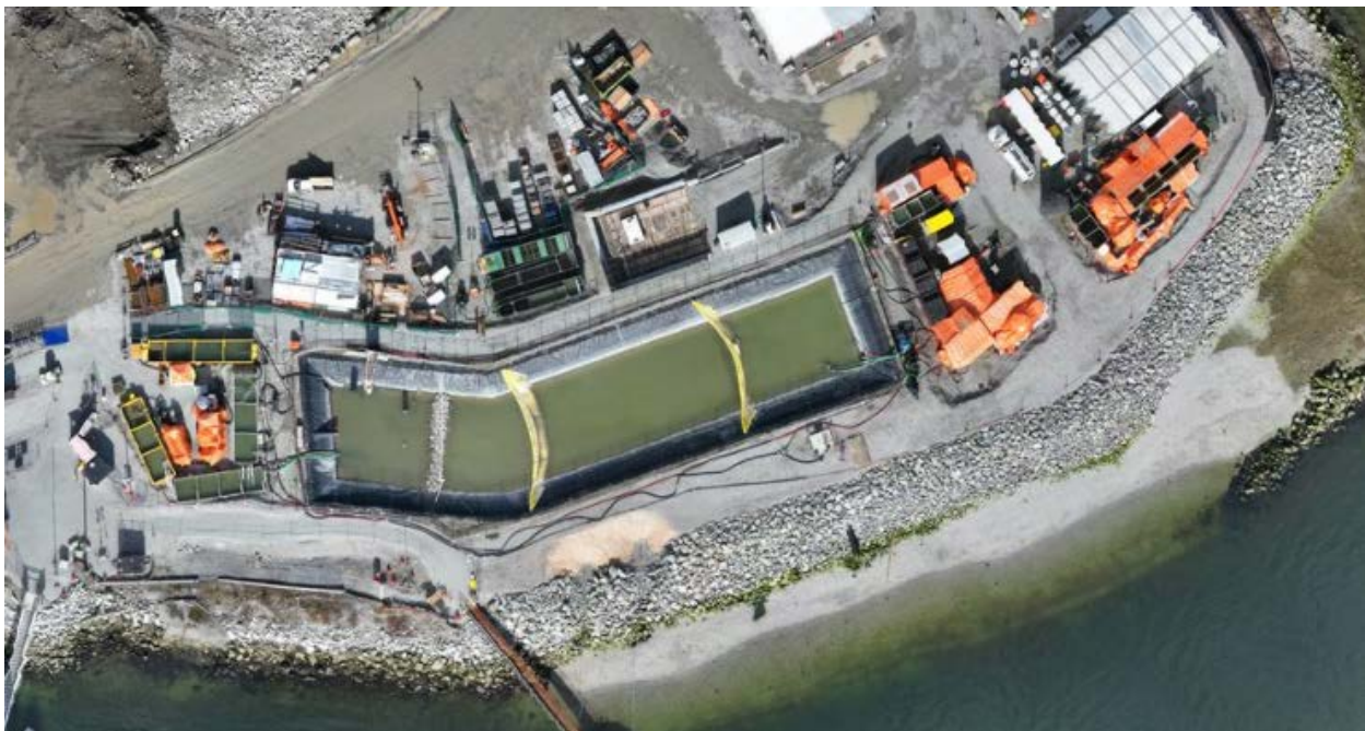
Figure 5: Aerial view of the West Sedimentation Pond (February 28, 2025). The TSS settling systems are located to the left (W500GPM) and right (ESC) of the pond.
