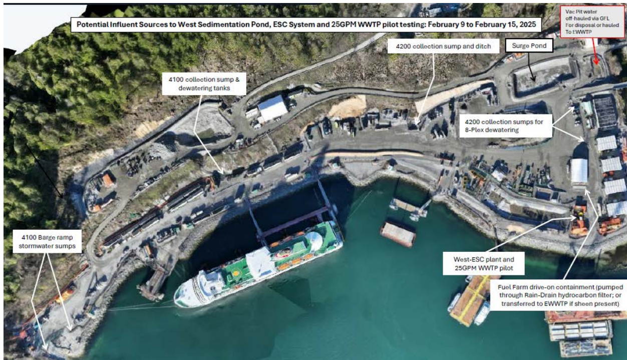
Figure 3: West Catchment contact water management facilities (February 9 – February 15).
