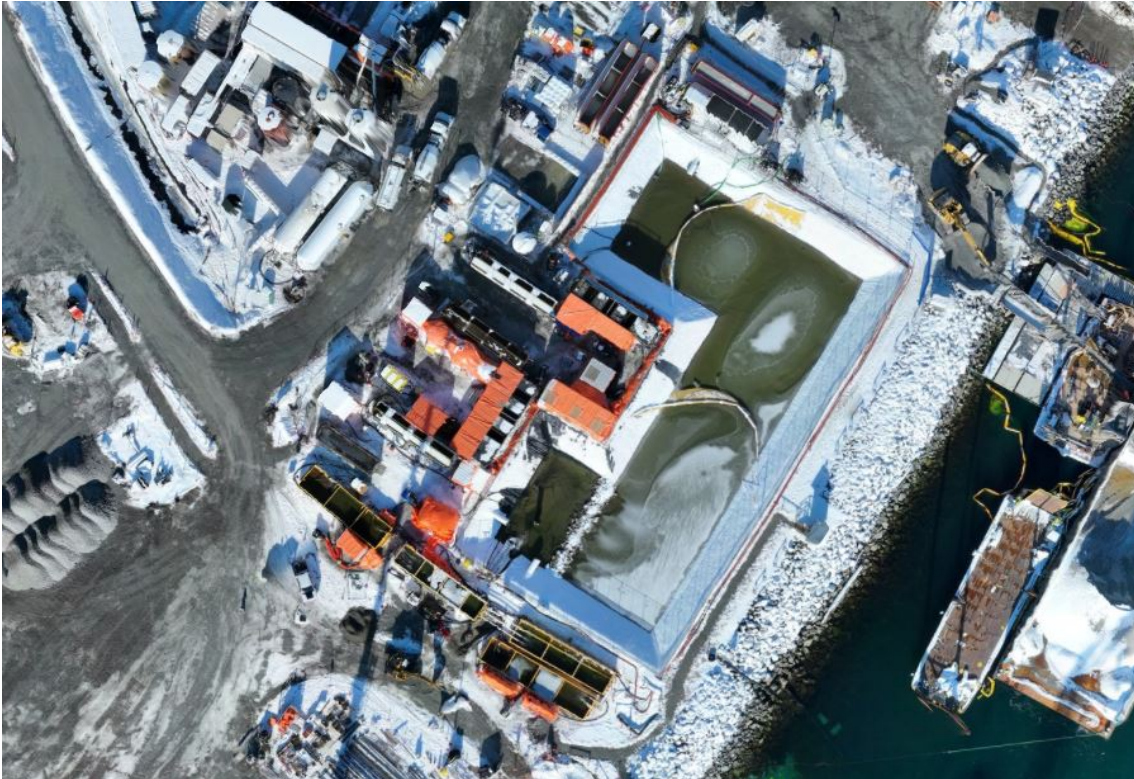
Figure 4: Aerial view of the East Sedimentation Pond (February 7, 2025). The East WWTP is located on the left side and the E500GPM TSS settling system is situated along the bottom edge of the pond.
