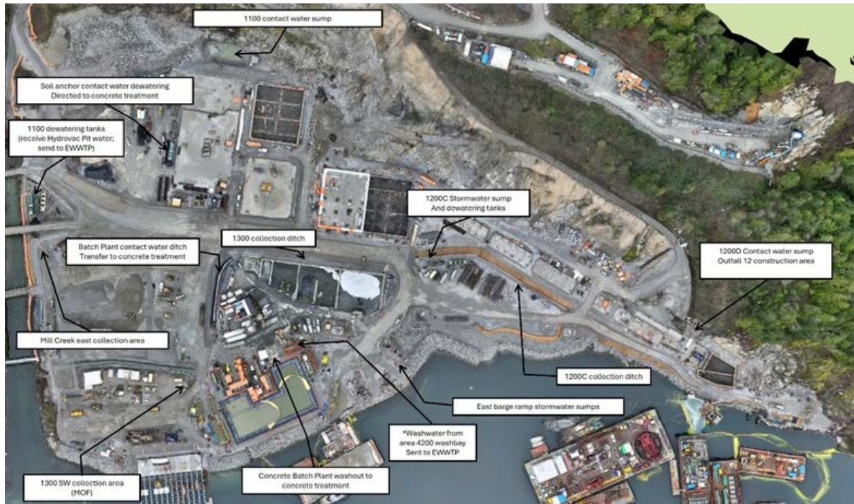
Figure 2: East Catchment contact water management facilities (January 12 – 18).
