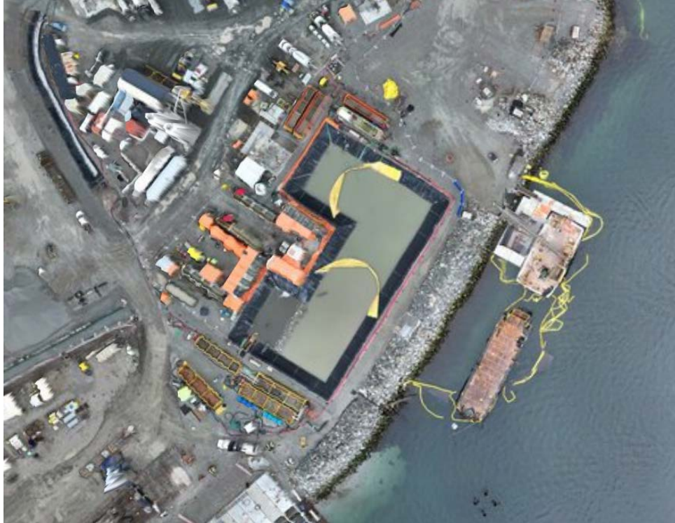
Figure 4: Aerial view of the East Sedimentation Pond (January 13, 2024). The East WWTP is located on the left side and the E500GPM TSS settling system is situated along the bottom edge of the pond.
