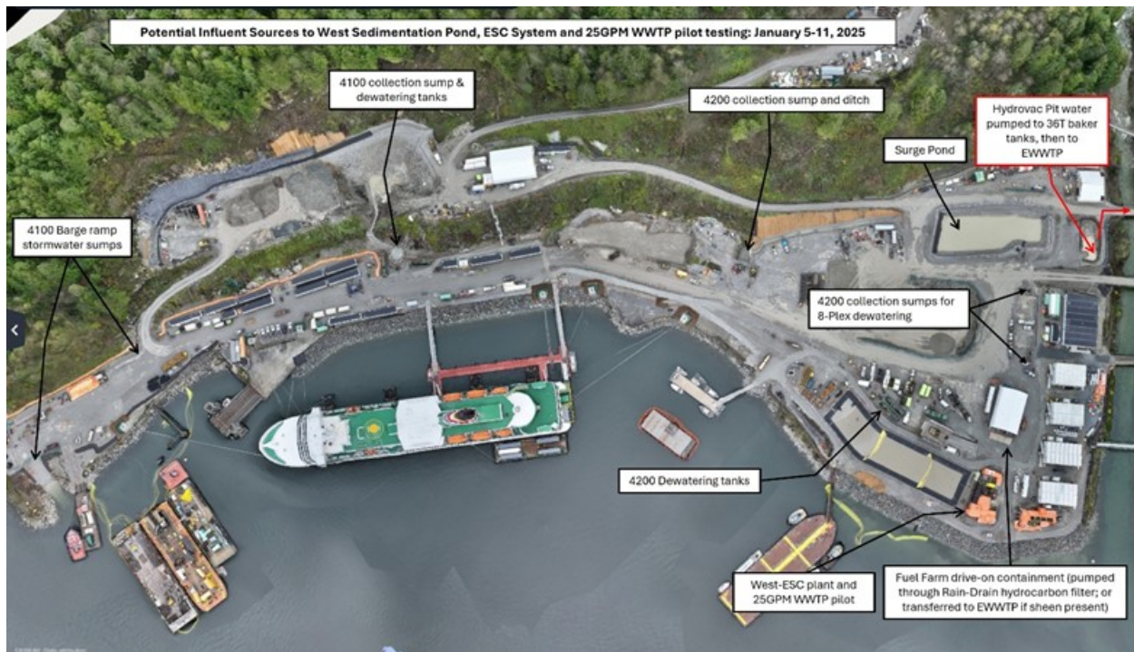
Figure 3: West Catchment contact water management facilities (January 5 – 11).
