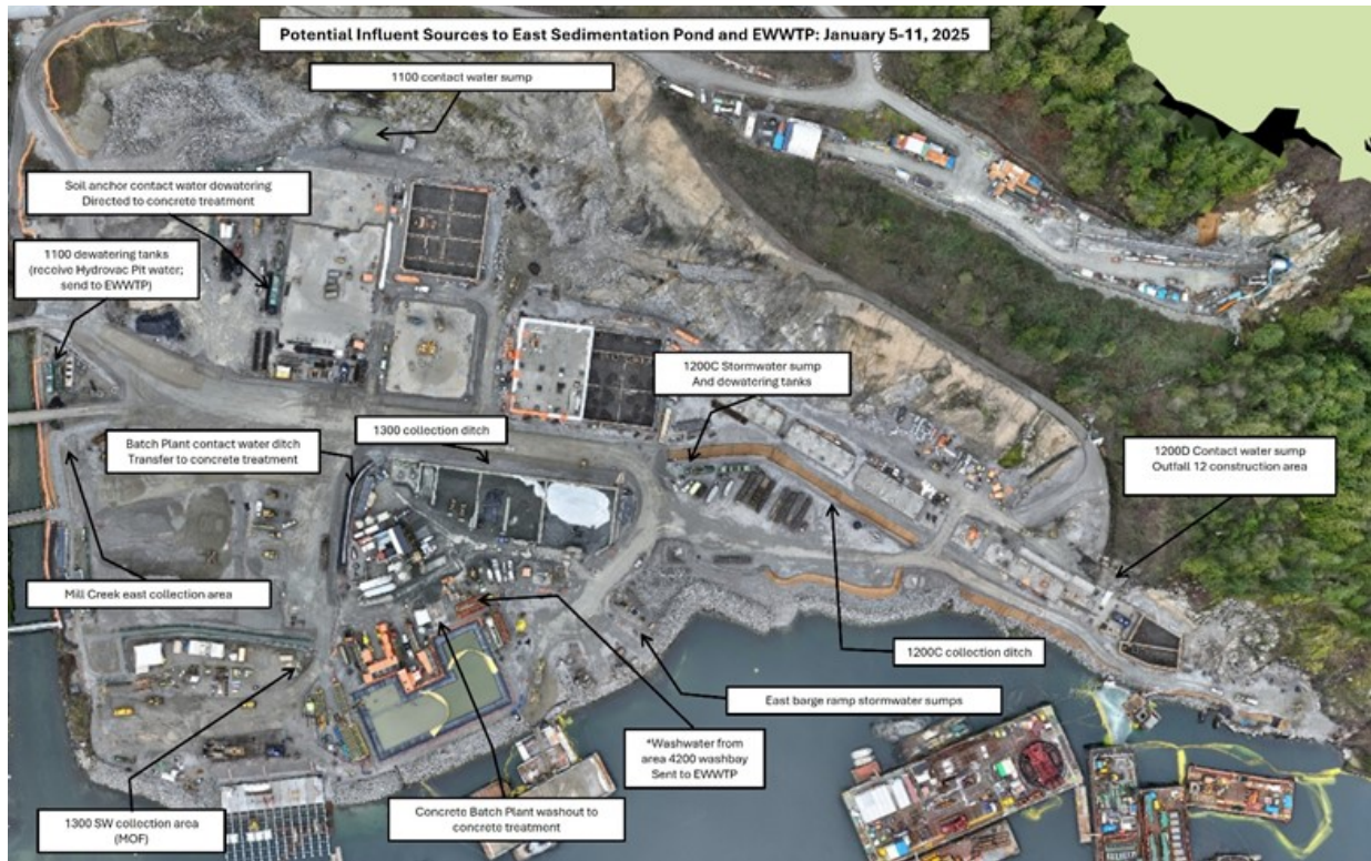
Figure 2: East Catchment contact water management facilities (January 5 – 11).
