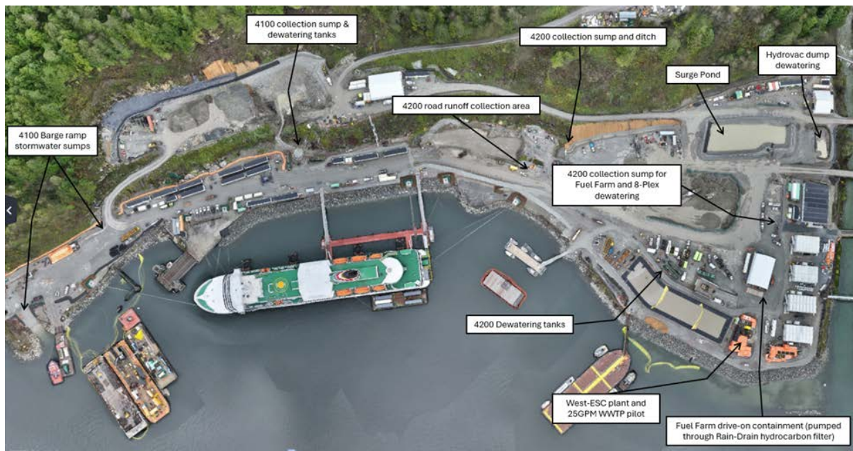
Figure 3: West Catchment contact water management facilities (December 15, 2024 – January 4, 2025).
