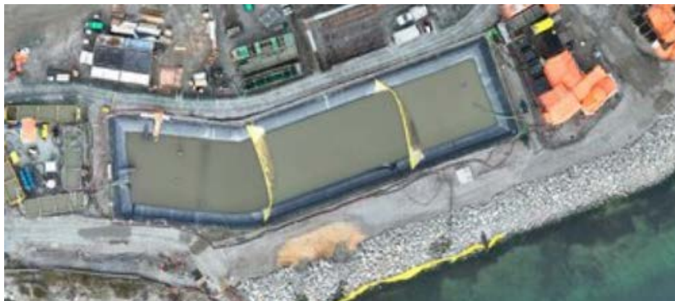
Figure 5: Aerial view of the West Sedimentation Pond (December 12, 2024). The TSS settling systems are located to the left (W500GPM) and right (ESC) of the pond.
