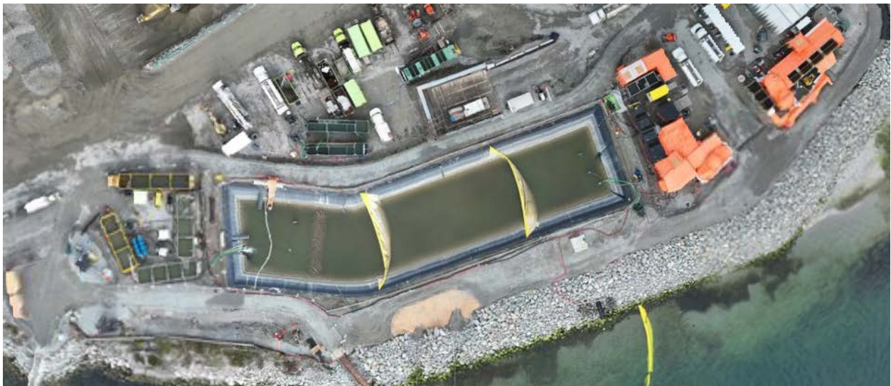
Figure 5: Aerial view of the West Sedimentation Pond (November 27, 2024). The old and new TSS settling (ESC) systems and the West WWTP are located to the right of the pond.
