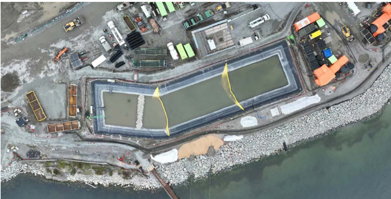
Figure 5: Aerial view of the West Sedimentation Pond (November 7, 2024). The TSS settling system (ESC System) and the West WWTP are located to the right of the pond.
