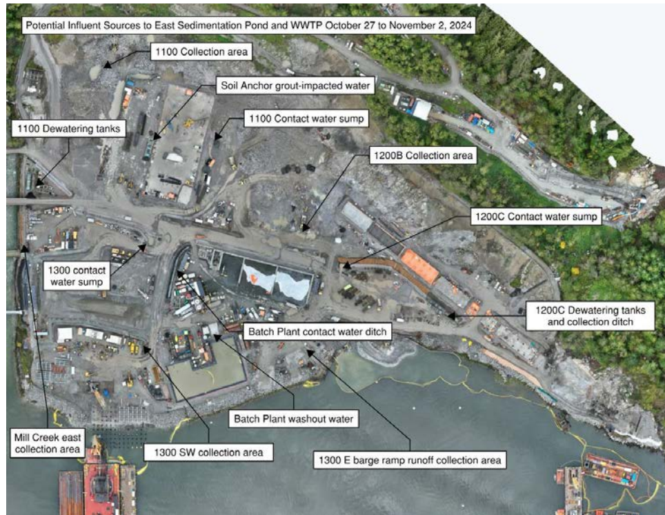
Figure 2: East Catchment contact water management facilities (October 27 – November 2).
