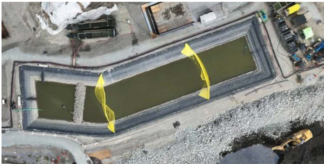
Figure 5: Aerial view of the West Sedimentation Pond showing the placement of two sediment curtains (September 13, 2024). The West WWTP is located on the right side of the pond.
