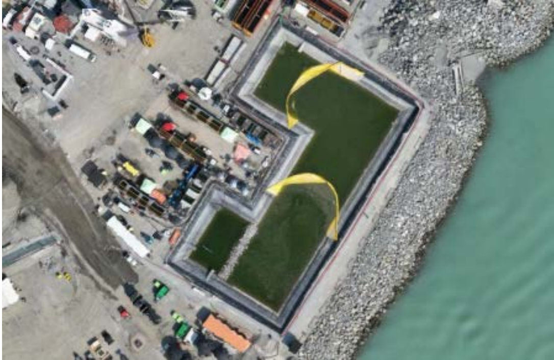
Figure 4: Aerial view of the East Sedimentation Pond showing the placement of two sediment curtains (August 9, 2024). The East WWTP is located on the left side of the pond.
