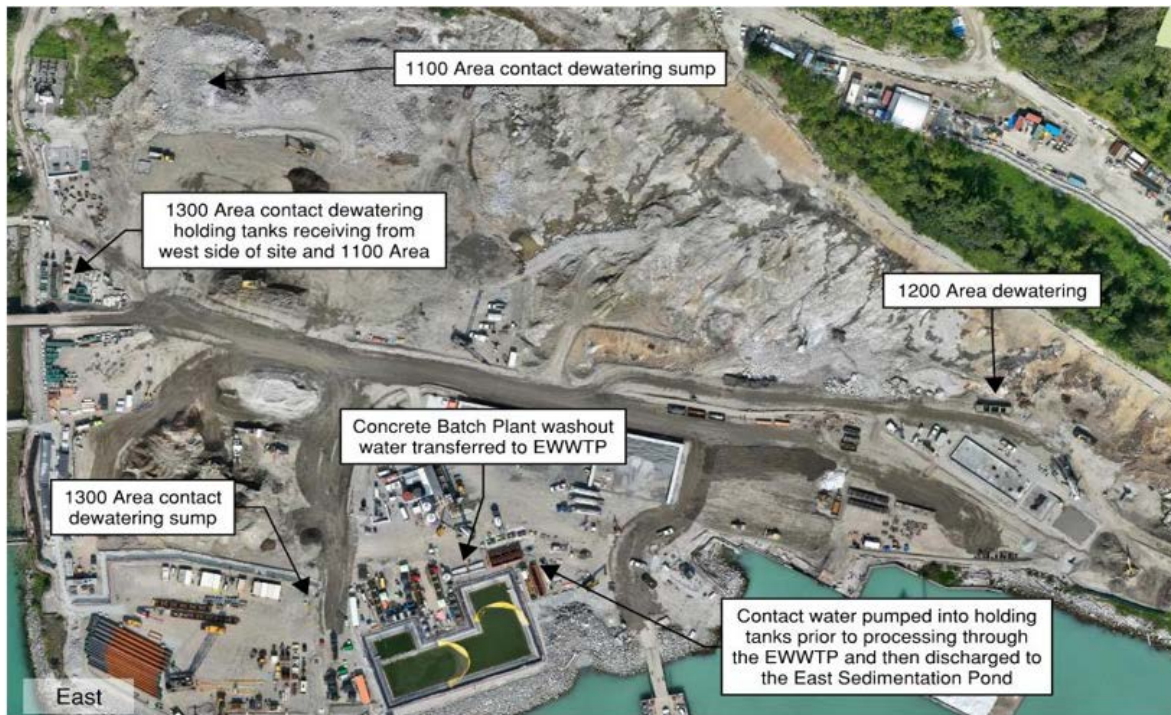
Figure 2: East Catchment dewatering areas. Potentially contaminated contact waters from the 1100 excavation and small amounts of concrete wash water were directed to the East WWTP for the August 4 – 10, 2024 monitoring period.
