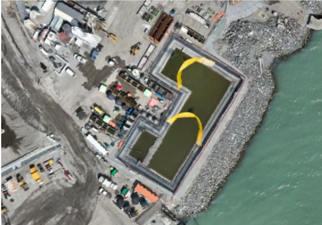
Figure 4: Aerial view of the East Sedimentation Pond showing the placement of two sediment curtains (July 26, 2024). The East WWTP is located on the left side of the pond.
