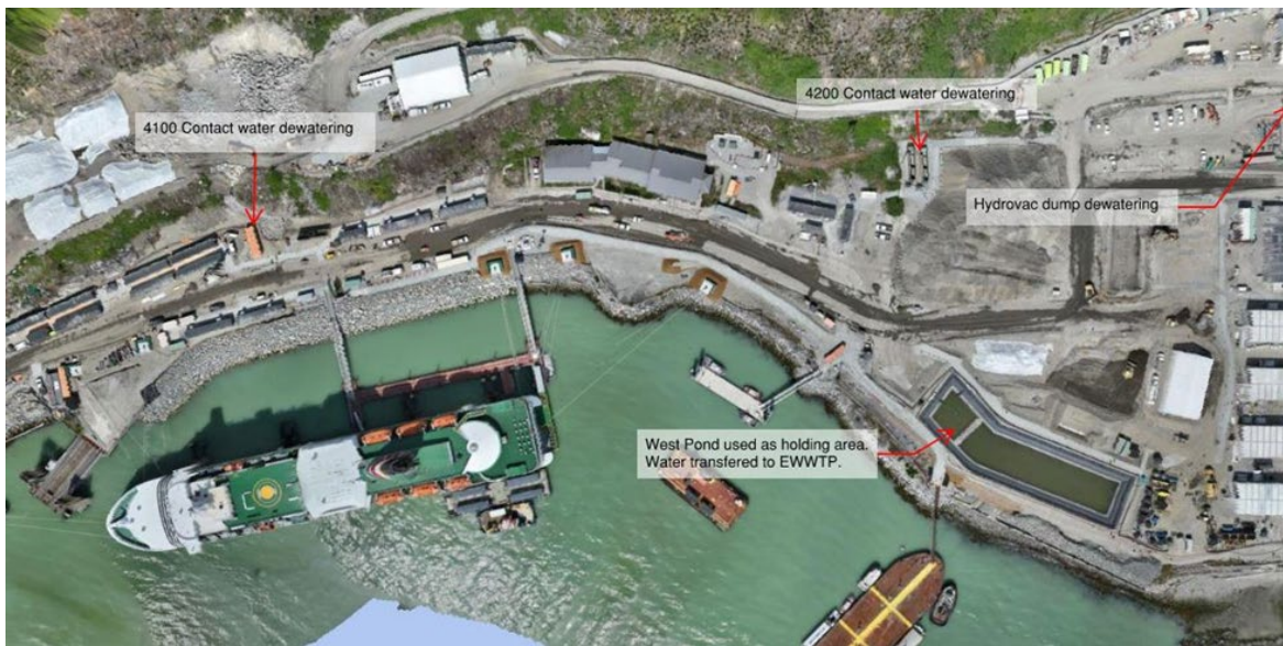
Figure 3: West Catchment dewatering areas. Dewatering of the West Catchment did not occur during the July 21 – 27, 2024 monitoring period.
