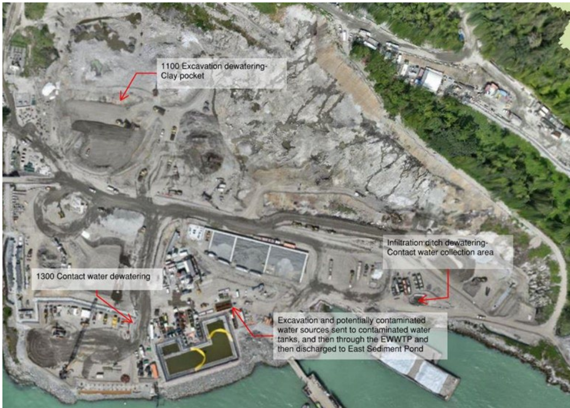
Figure 2: East Catchment dewatering areas. For the July 21 – 27, 2024 monitoring period dewatering was only active for the 1100 Excavation and was directed to the East WWTP.
