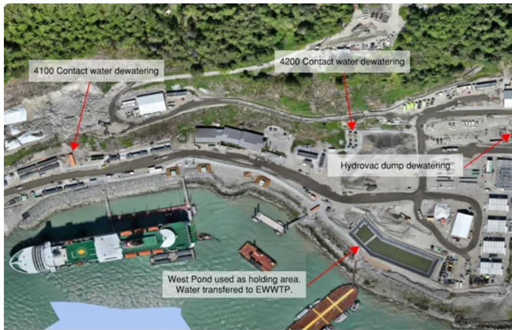
Figure 3: West Catchment Areas Dewatered to the East WWTP July 14 – 20, 2024.
