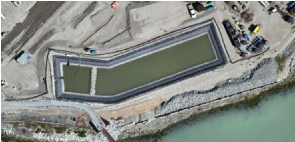
Figure 5: Aerial view showing the West Sedimentation Pond and West WWTP (located to the right of the pond) on July 12, 2024.
