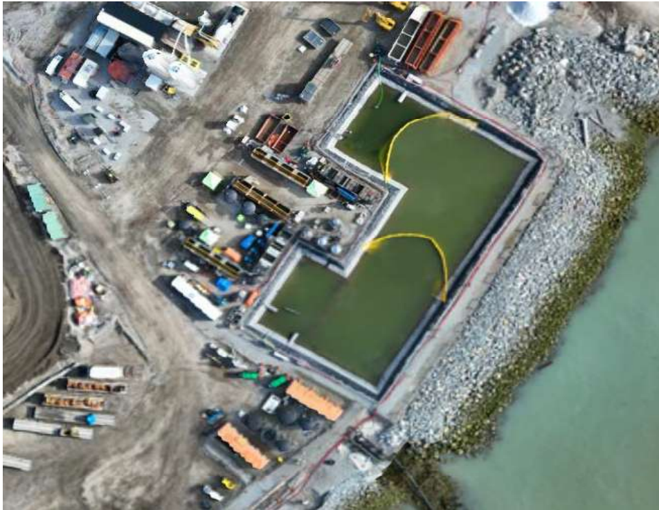
Figure 2: Aerial view of the East Sedimentation Pond showing the placement of two sediment curtains (July 2, 2024). The East WWTP is located on the left side of the pond.
