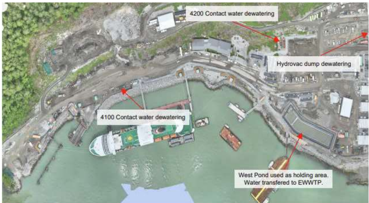
Figure 3: West Catchment Areas Dewatered to the East WWTP June 23 to June 29.
