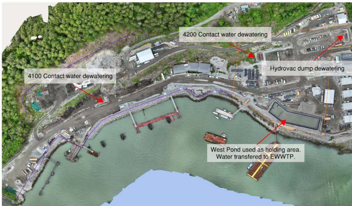
Figure 3: West Catchment Areas Dewatered to the East WWTP June 9 to June 15.
