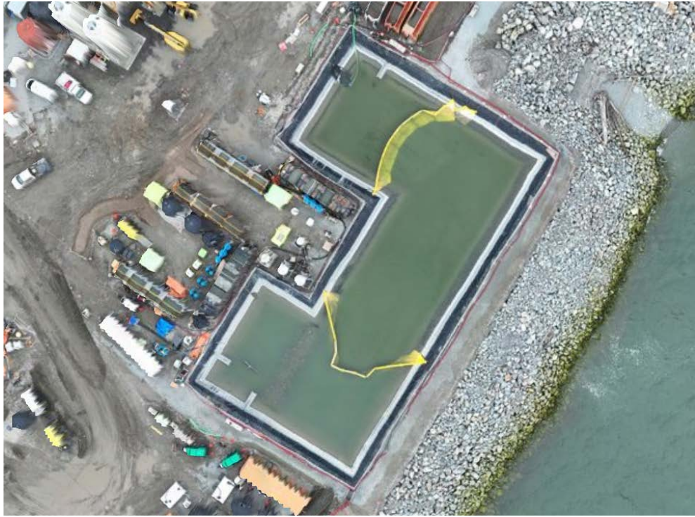
Figure 2. Aerial view of the East WWTP and East Sedimentation Pond (May 25, 2024).
