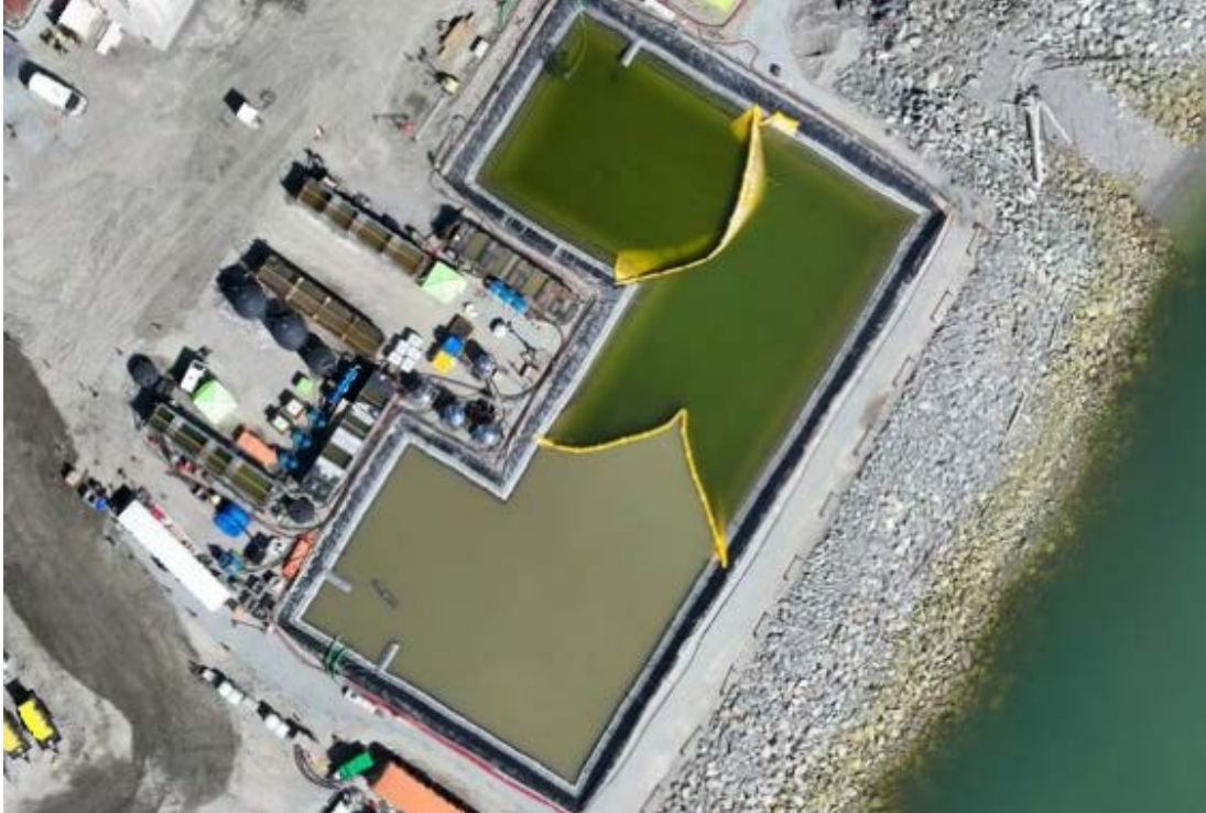
Figure 2. Areal view of the East WWTP and East Sedimentation Pond showing the placement of two sediment curtains. Water at the inlet (southwest) section of the pond is cloudy due to elevated TSS in the influent. A progression to less turbid water is observed in the sediment curtain cells from the pond inlet (bottom centre of photo) to the outlet (top centre of photo) (May 10, 2024).
