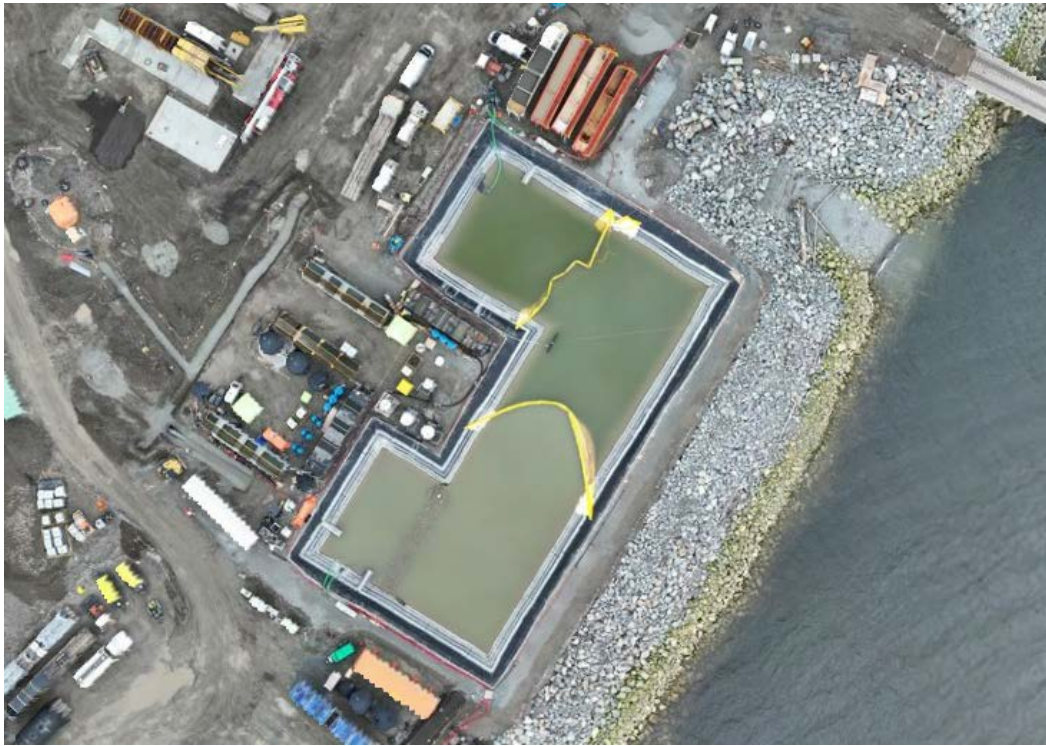
Figure 2: Areal view of the East WWTP and East Sedimentation Pond showing the placement of two sediment curtains. Water at the inlet (southwest) section of the pond is brown due to elevated TSS in the influent. A progression to less turbid water is observed in the sediment curtain cells from the pond inlet (southwest corner) to the outlet (northern corner) (April 24, 2024).
