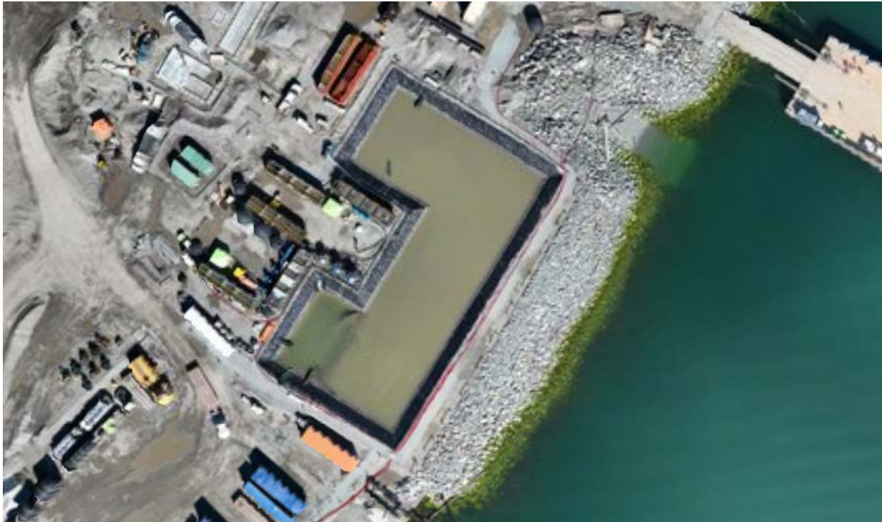
Figure 2. Areal View of the East WWTP and East Sedimentation Pond (April 5, 2024).
