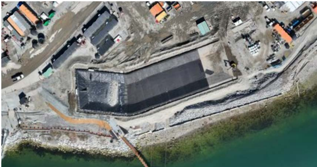
Figure 3: Areal view of the West Sedimentation Pond Construction Progress (April 5, 2024).
