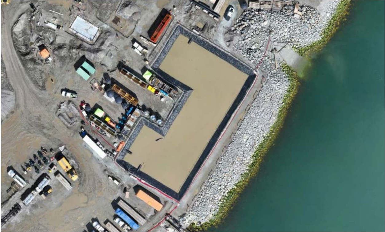
Figure 2. Areal View of the East Sedimentation Pond and Wastewater Treatment Plant (29 March 2024)
