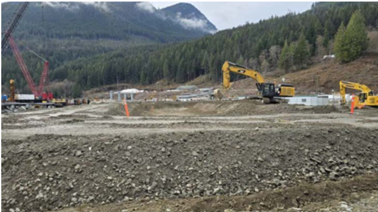
Figure 3: West Sedimentation Pond berm placement (23-Mar-2024).
