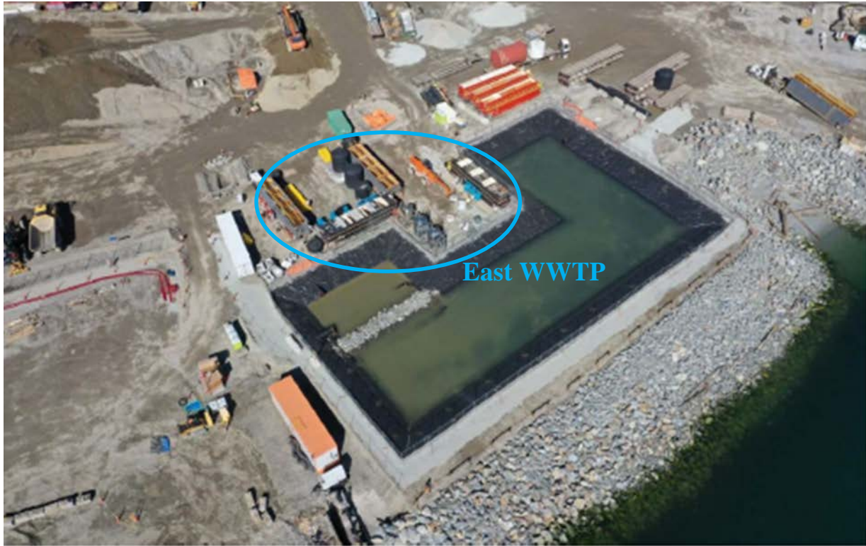
Figure 2: Areal view of the East Sedimentation Pond and the partially assembled East Wastewater Treatment Plant (East WWTP) near the centre of the photo (17- Mar-2024).
