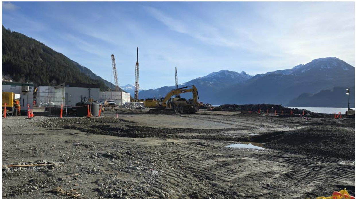
Figure 3: West Sedimentation Pond site levelling and sub-grade preparation (14- Mar- 2024).
