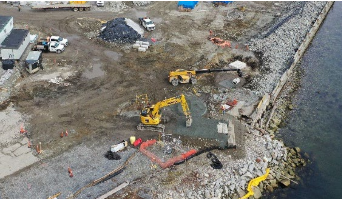
Figure 3: West Sedimentation Pond site preparation and construction (06-Mar-2024).
