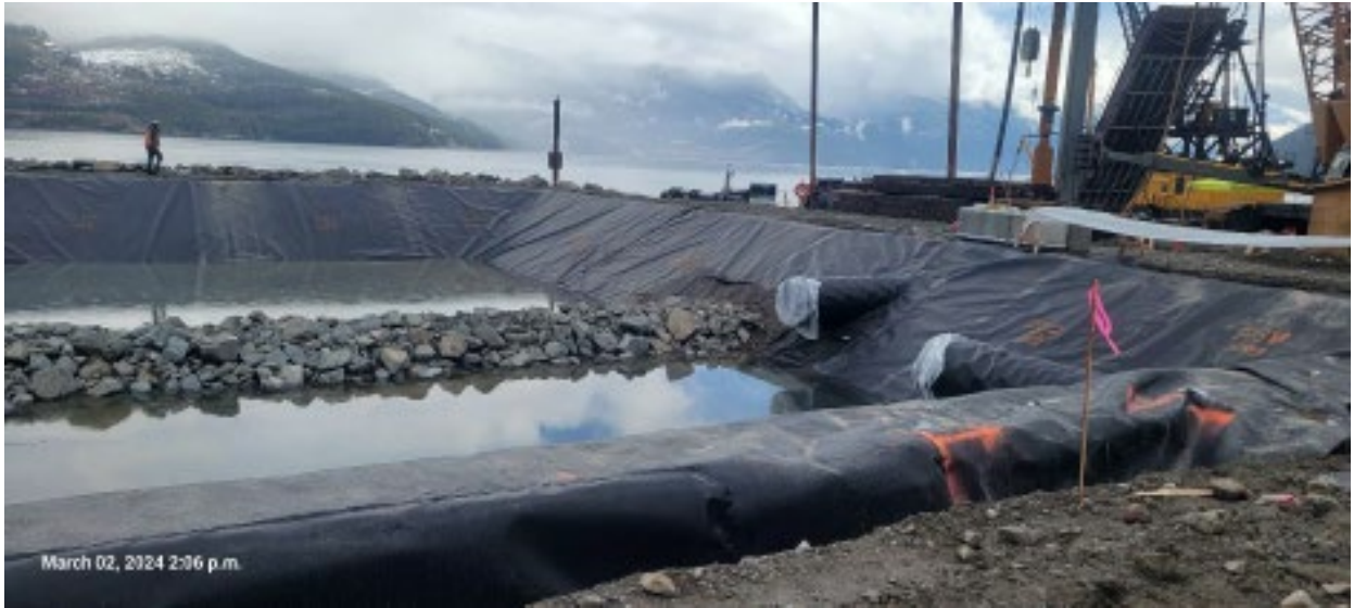
Figure 1. East Sedimentation Pond showing placement of the inlet pipes (02-Mar-2024).
