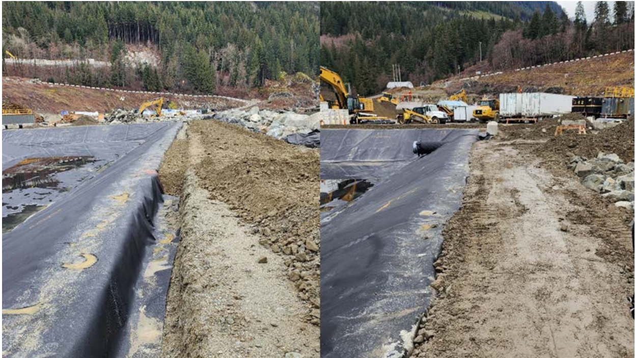
Figure 1. Backfilling the East Sedimentation Pond liner key trench (23-Feb-2024)
