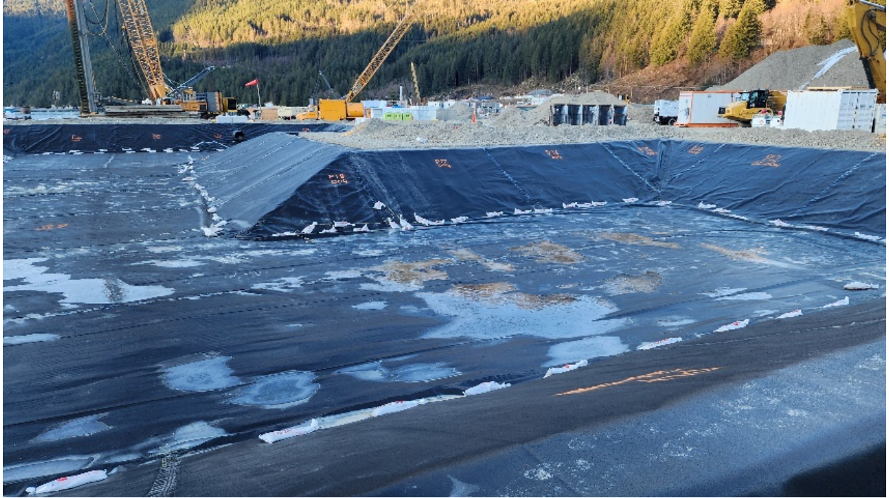
Figure 1. East Sedimentation Pond showing placement of the liner (16-Feb-2024).
